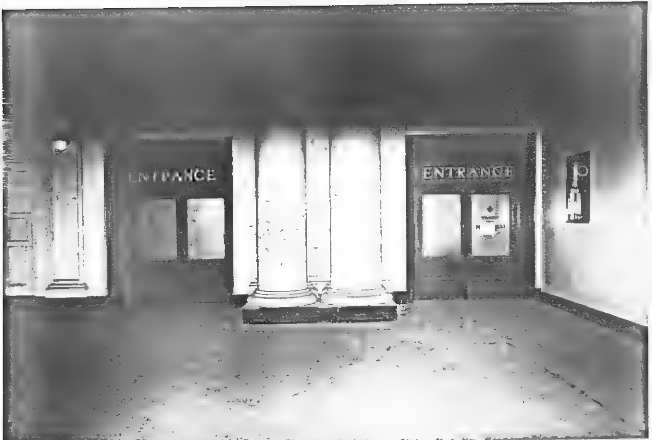
Typical view of paired pilasters of ferry concourse, which occur at the beams of the skylight areas of upper floor (other paired groupings have been removed).
